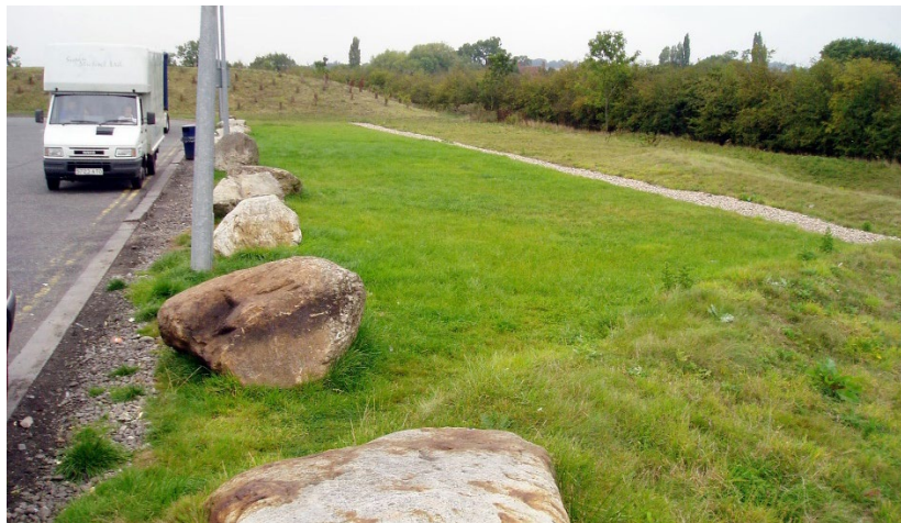
Figure 14: Example of filter strips (Source: Susdrain)
